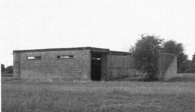
Magazine with removed earth bank.
